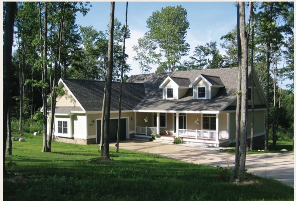
A modern design home spotlighting exquisite expressions created by Bob Fate Builder, Inc. The covered front porch consists of a beaded ceiling of Douglas fir, Brazilian Red Wood decking and fiberglass railing. The home, constructed with Insulated Concrete Forms, giving an R-50 insulation value, and maintenance free Fiber Cement siding, result in numerous long term rewards of energy efficiency.
